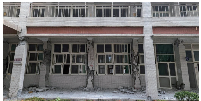
(b) Complex building (not seismically retrofitted)
