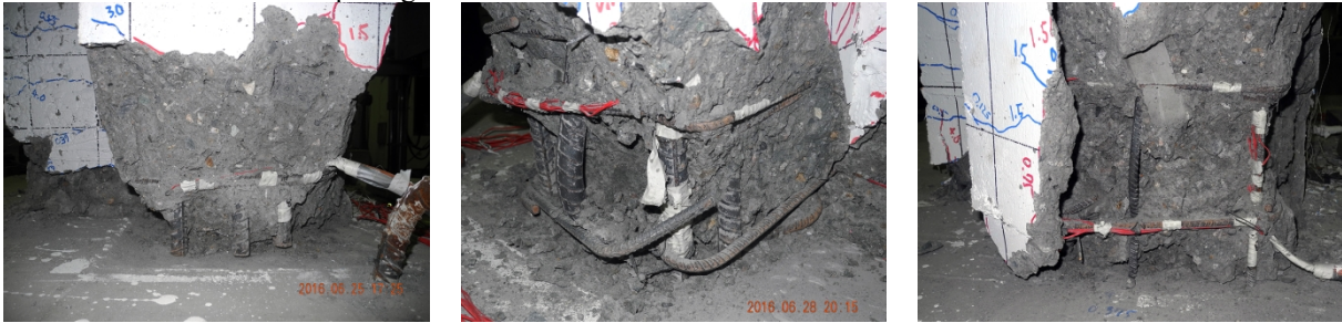
Closing of the interface between the column and foundation
